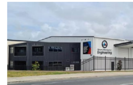
Right: Mount Maunganui Engineering in Lot 6.
